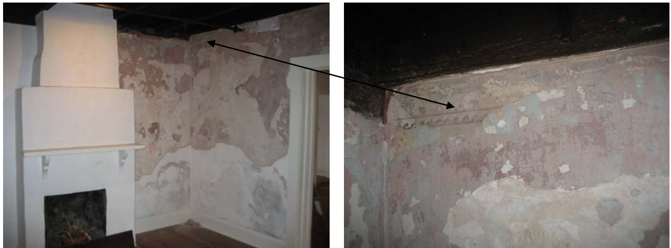
Room 204, south east corner, large fragments of a c. late 19 th c. wallpaper border that was recently revealed when the walls were scraped, thus removing later paints and skim coats of plaster.
