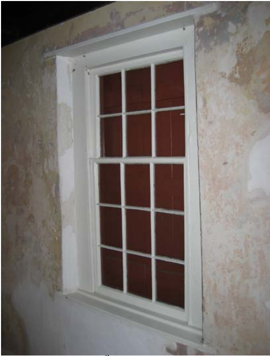
Typical late 19 th c. sashes in window 205
