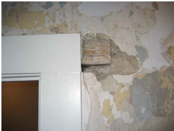
Room 200, Doorway 200-B, upper right side of frame showing exposure of original header after removal of old plaster that covered it. The wood header shows one layer of very old white whitewash.
