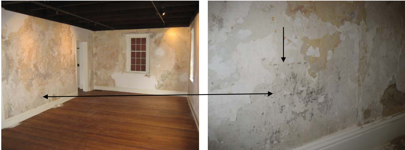
Room 200, Arrows point to vestiges of a ca. mid-19 th c. black painted wainscot that extended up to 20" from floor.
