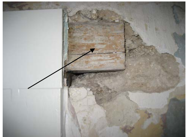
Room 200, Doorway 200-B, upper right side of frame showing exposure of original header after removal of old plaster that covered it. The wood header shows one layer of very old white whitewash.
